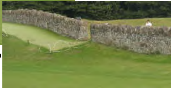
Now – That's a hazard
